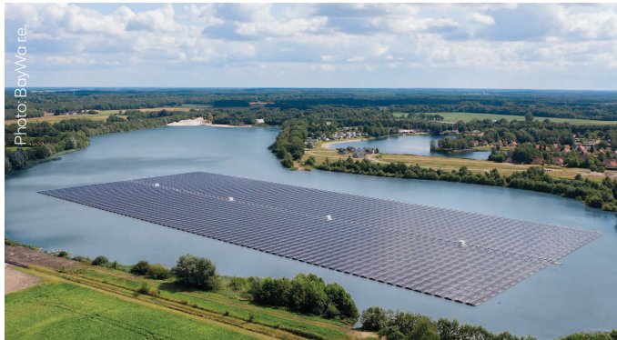
Floating solar makes use of unused bodies of water
