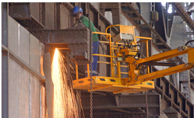
Molten metal slag can ignite surfaces many stories below
