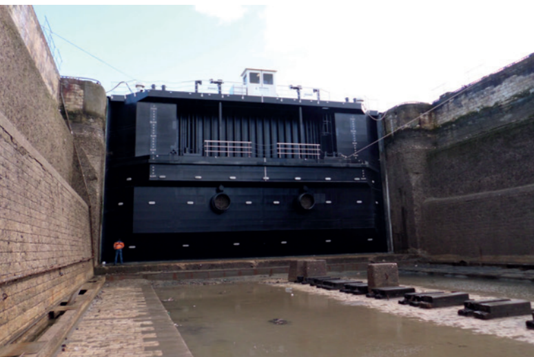
Chatham Docks Caisson Lock Gates - www.ravestein.nl
