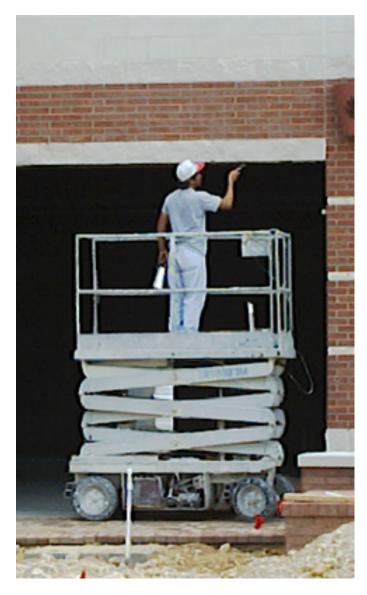
Scissor lifts provide a safe and reliable platform for workers to perform job tasks when used according to the manufacturer's instructions. When not used properly, scissor lifts can present a serious hazard to workers. Employers are responsible for keeping workers safe. This Hazard Alert highlights specific hazards present in workplaces where scissor lifts are used and controls employers must implement to prevent injuries or fatalities
