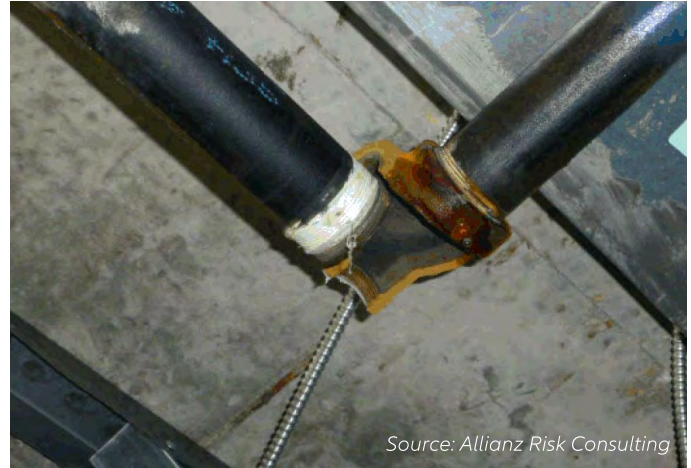
Fractured pipe fitting
