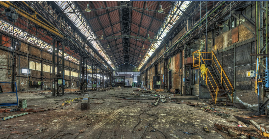
Large abandoned industrial hall
