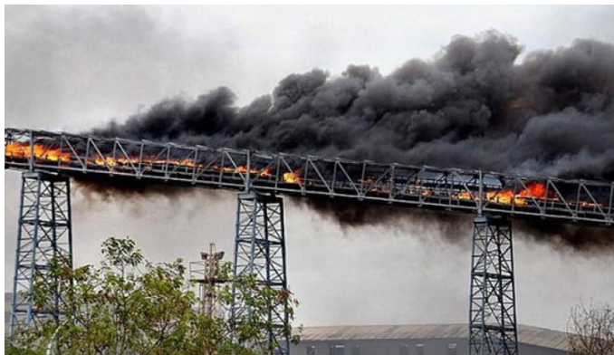
Conveyor belt on fire
