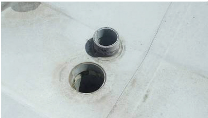
Conventional roof drainage system Siphonic roof drainage system
