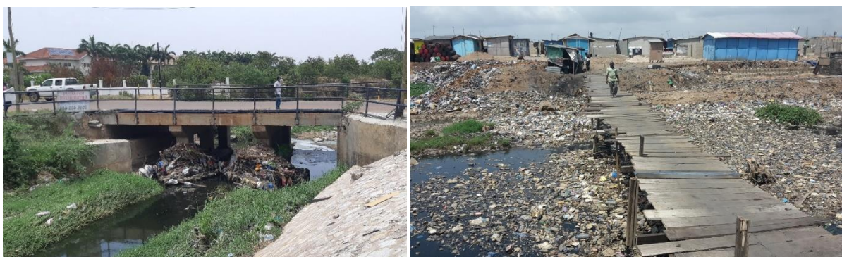
Figure 37: Examples of waste accumulated in drains. Source: Fotos by Dorien Lugt (HKV) (Left) and Durk Klopstra (HKV) (Right).
