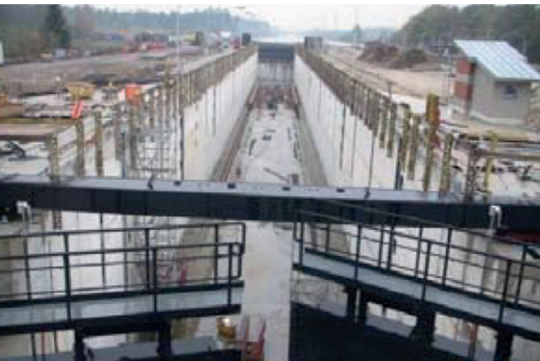
Shock absorber beam in front of mitre gates - Google
