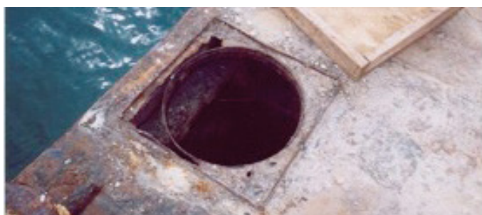
Manhole covered with wooden hatch.
