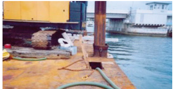
Note hole cut in deck and the portable pump & hose on deck. Barge must be regularly pumped to keep the compartment from flooding.
